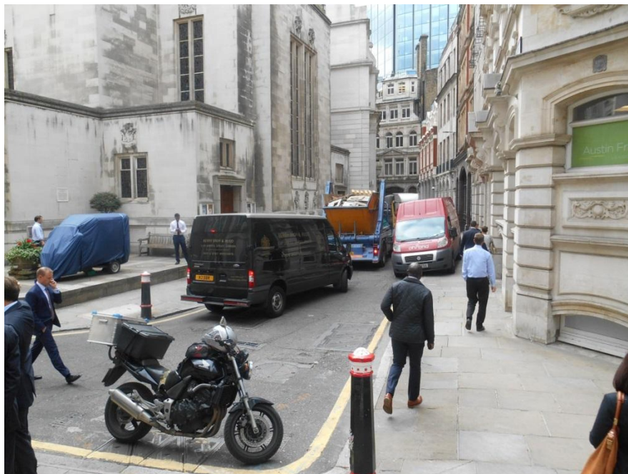
Austin Friars Central Section – Before works
